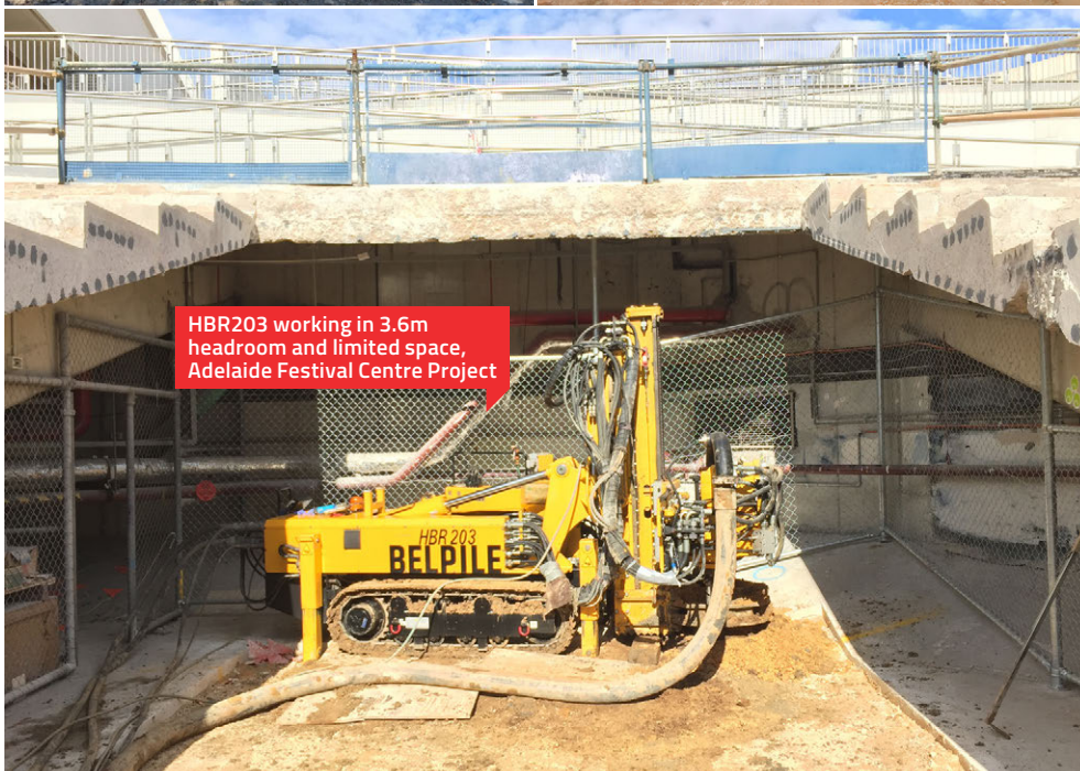
Mobilisation/ setup of limited access machinery
