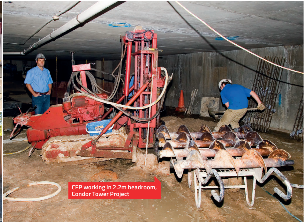
Mobilisation/ setup of limited access machinery
